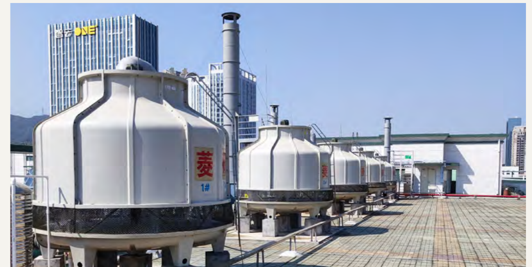
Balancing pipes for cooling towers
